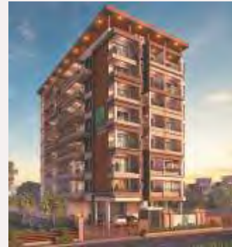
Inland Apeiron Near Bunts' Hostel, Pinto's Lane, Mangaluru
