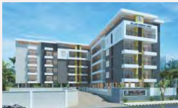
Inland Buenos Aires (Res) Lobo Lane, Bendoor, Mangaluru
