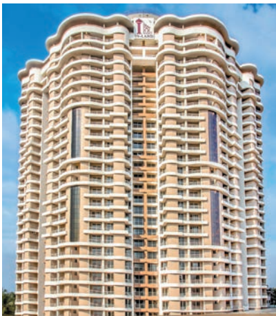
Inland Windsors (Res) Airport Road, Mary Hill, Mangalore
